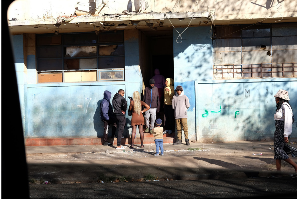
Hillbrow, Johannesburg, where the hijacking of buildings is a major urban challenge. As of 2026, at least 188 properties in the city centre had been hijacked. Photo supplied
