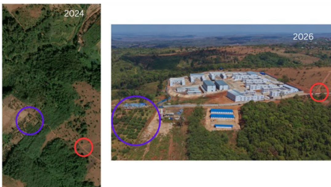
Land in the Laoka area has been rapidly reorganized around the scam industry, with a compound of some 30 buildings built in roughly a year. Images: Apple Maps satellite image 2024 (left) and drone photograph February 2026 (right), with annotations by Kem Rathanak
