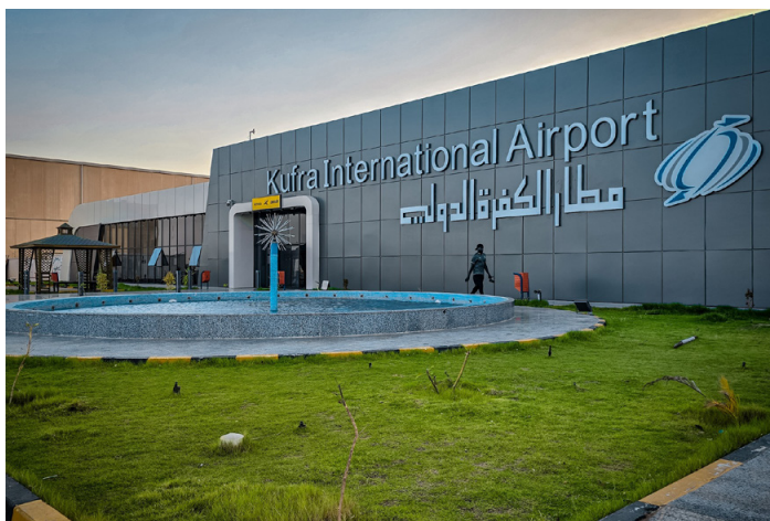
Kufra airport, after reported refurbishment by the LAAF's Land Forces, 2025. Photo: Facebook
