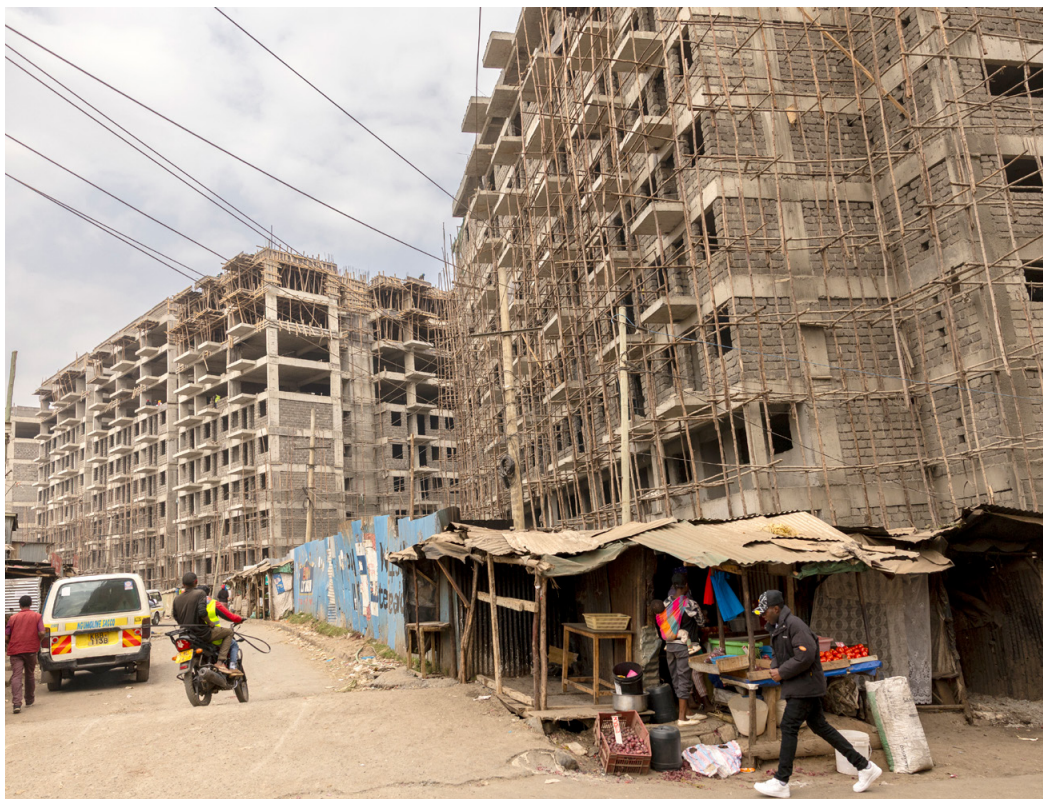
The construction industry in Africa has been identified as a major money laundering risk. © Simon Maina/AFP via Getty Images
