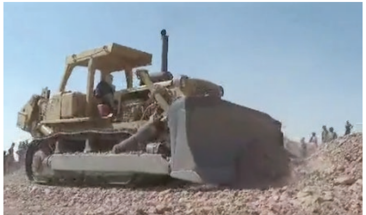
SONEMIC constructs roads in Kouri Bougoudi, November 2023.
