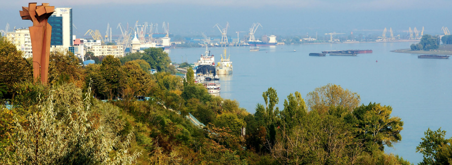
The port of Galați, Romania, has been upgraded to accommodate increased cargo traffic. © Ioan Cepaliga/Wikipedia
