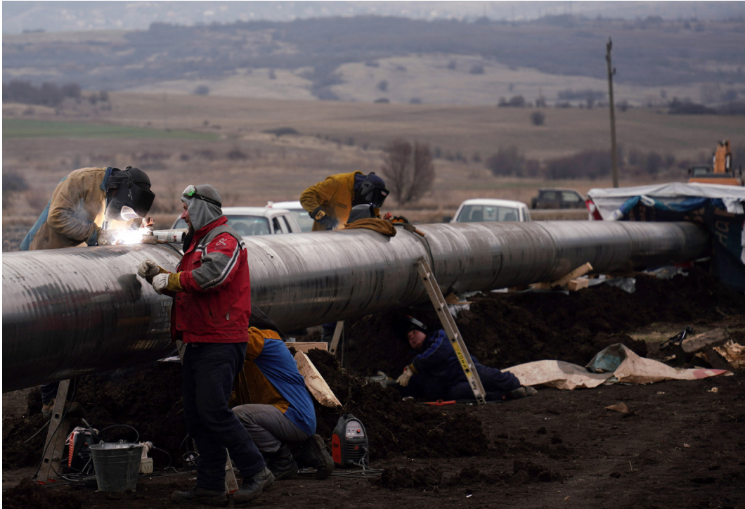
Bulgaria has begun work on a gas pipeline to neighbouring Serbia to reduce dependence on Russian flows.
