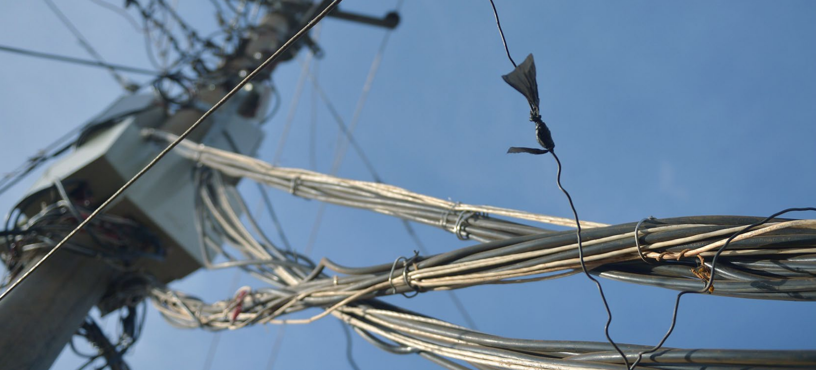
A wire denoted by a piece of polythene tied around it is used to make an illegal connection. Photo: Tony karumba/AFP via Getty Images
