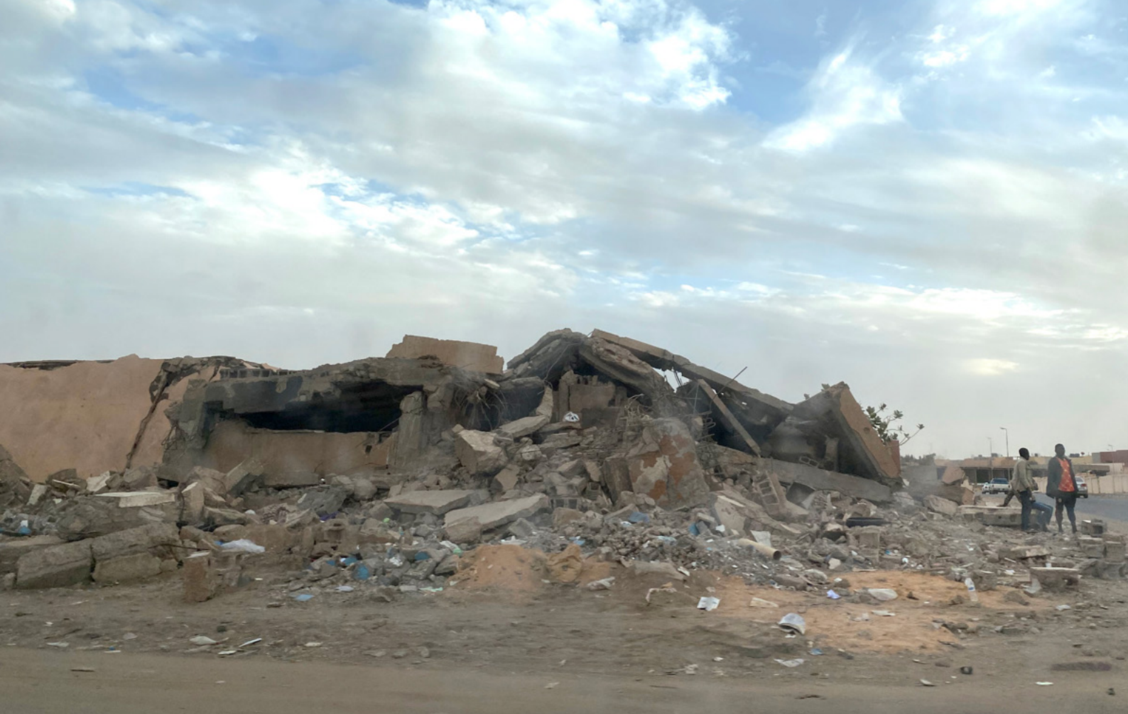
Bombed building in Sebha, January 2021.
