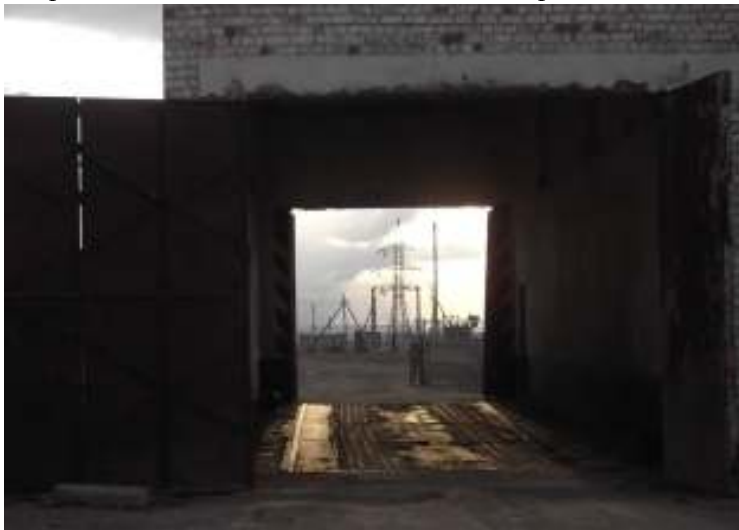
Figure 7: Unused Customs facilities at Torugart
