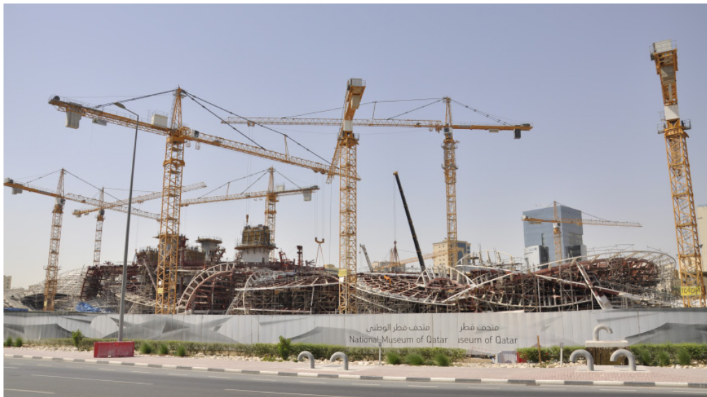
The National Museum of Qatar, an architecturally stunning undertaking, currently under construction in Doha. (Pygmalion Karatzas Photography).
